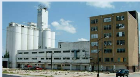
MFA Milling Facility (BEFORE)
